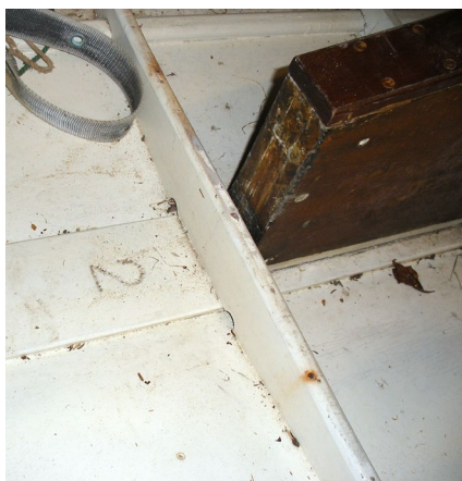
Floor boards out, and yes, it IS No 2!
